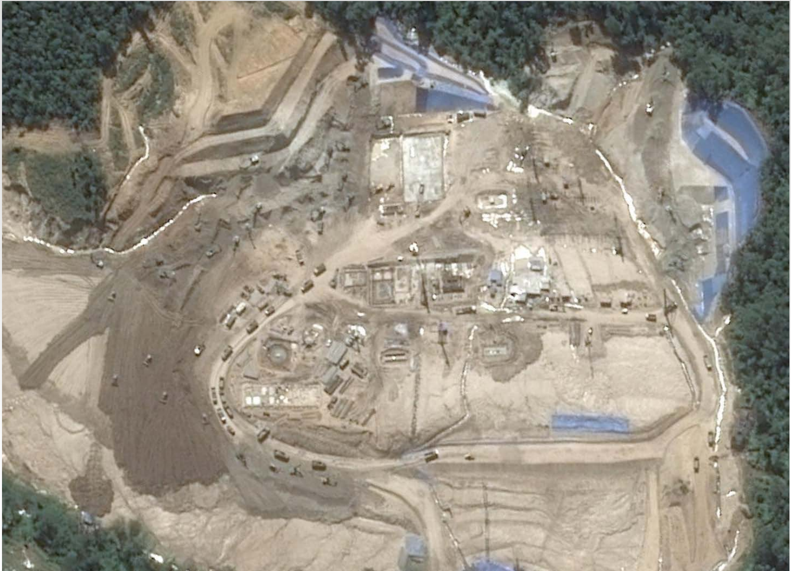
Site Condition after DCM Soil Improvement
