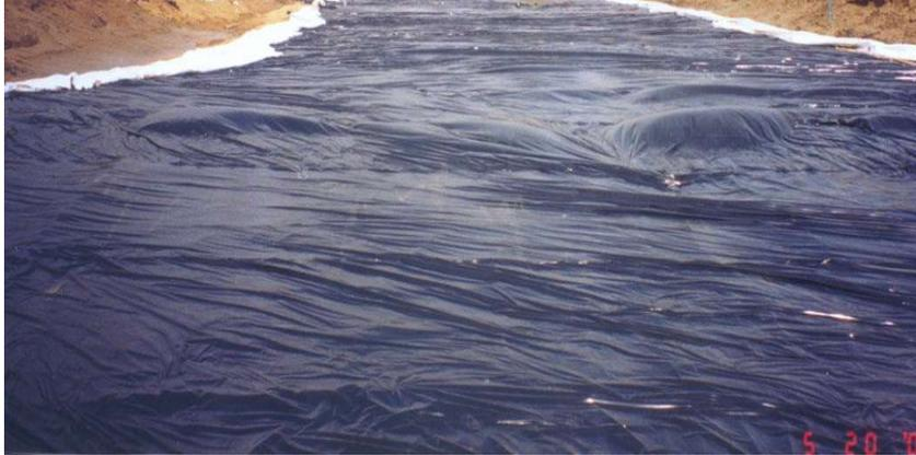
**Placement of a protection layer on top of the membranes**
